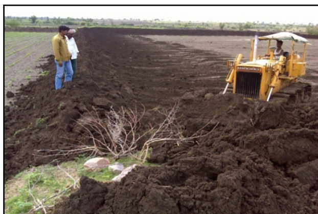
Bunding work in progress
