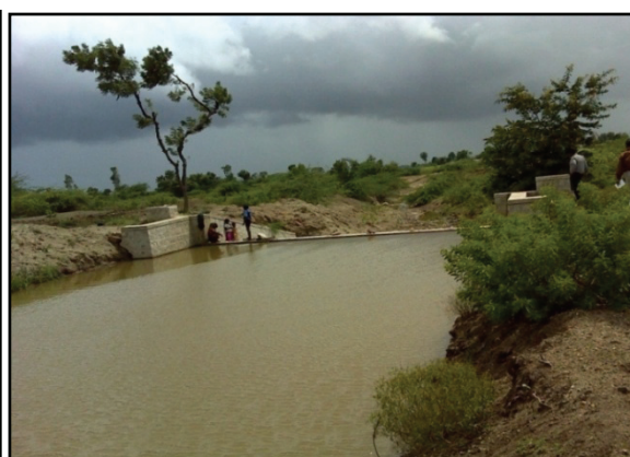
Check dam – Entry point Activities
