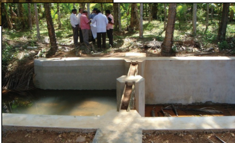
Entry Point Activity: Vented dam constructed in Manki Village, Sampolli SWS;Honnavaara taluk; Uttara Kannada district
