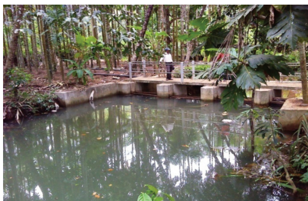
Vented Dam at Mavalli, Bhatkal taluk, UK District
