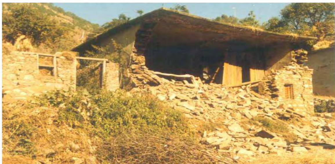
(a) Partial collapse of stone masonry walls during 1991 Uttarkashi Earthquake
