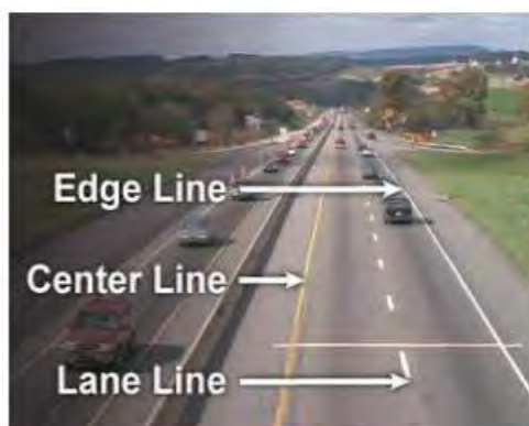
Figure 1: Road line markings
