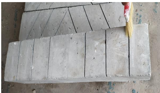
Fig. 4: Cleaning of groove
