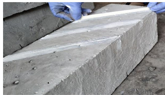
Fig. 5: Placing of GFRP
