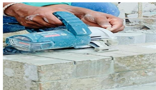
Fig. 3: Groove cutting
