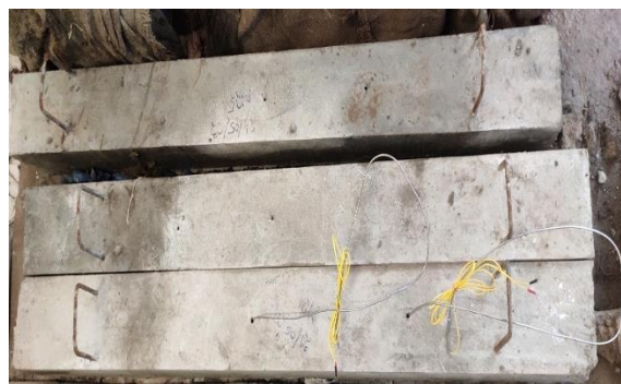
Fig2. Beams with sensors embedded within
