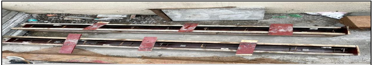
Fig 3. Shuttering for beams with post-cut opening
