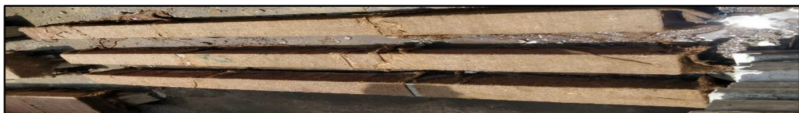
Fig 7. Curing of beams
