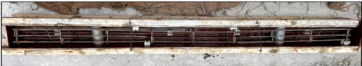
Fig 4. Shuttering for beams with pre-cut opening
