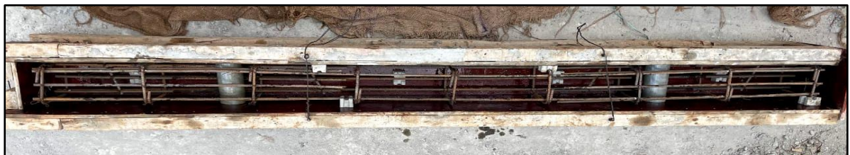
Fig 5. Casting of beams
