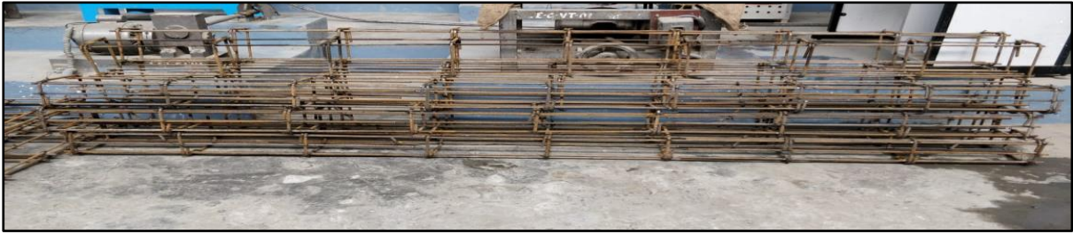
Fig 2. Bar bending of steel reinforcement
