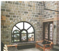
The walls of the house, built of stone, are based on a rat-trap design. The air is trapped between the two walls and acts as an insulator, controlling the room temperature.
